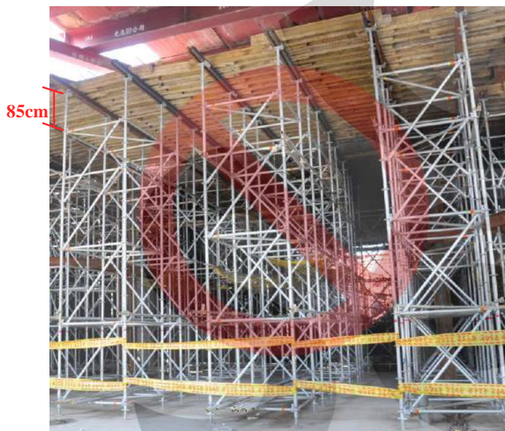
(8) The overhang is too long to keep safety load
