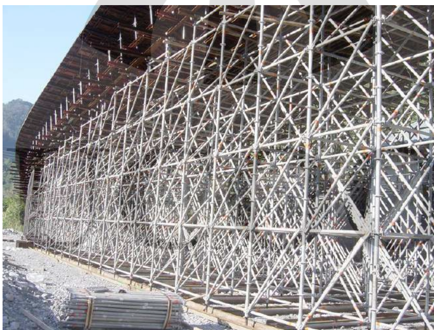
(7) Diagonal configuration in the same direction.
