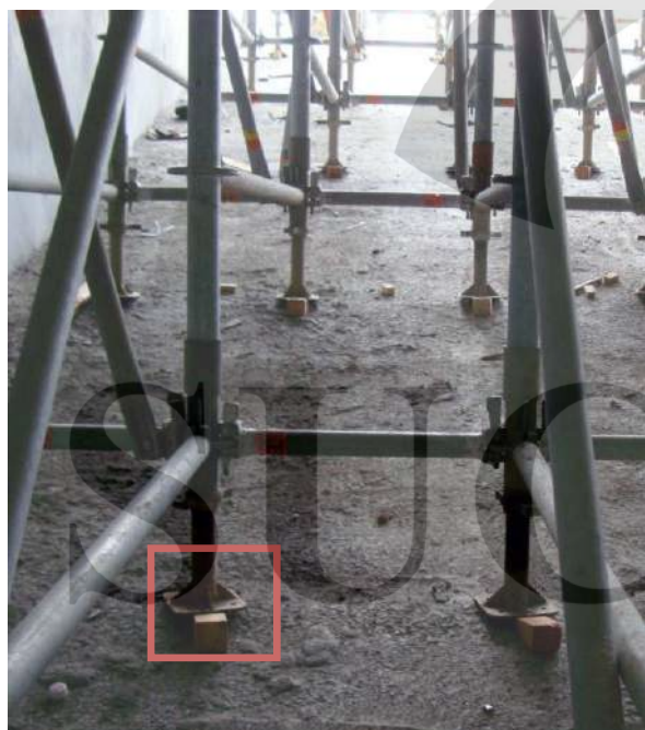
(14) Use the triangle chuck below the Jack Base on slope.
