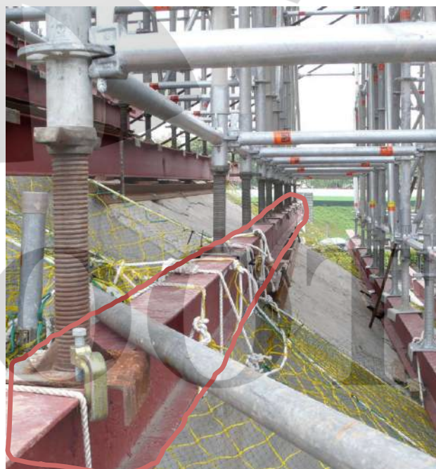
(15) Use the H beam on the slope
